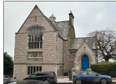
Fig. 2. Church House, Armagh.
