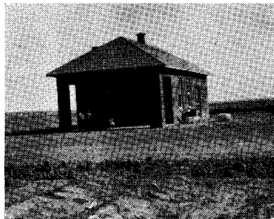
Fig. 4.-Office Building (1913). Used until 1948.
