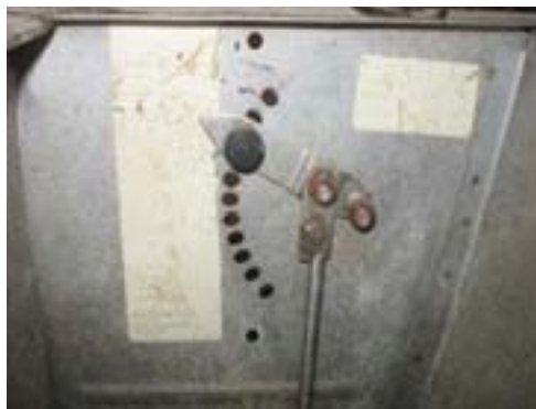
Figure 1. Example of STACO stainless steel dry feeder on feeder setting 3.
